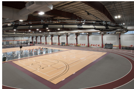
Alvernia University, Reading, PA. Draper Smart Gym control system. Photo: Alan Wycheck.
